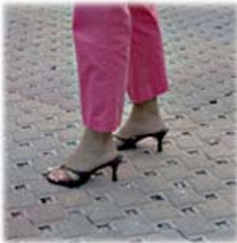
**A:** Solid pavers can be introduced into PICP paving patterns in pedestrian areas to accommodate a variety of shoes including high heels.
