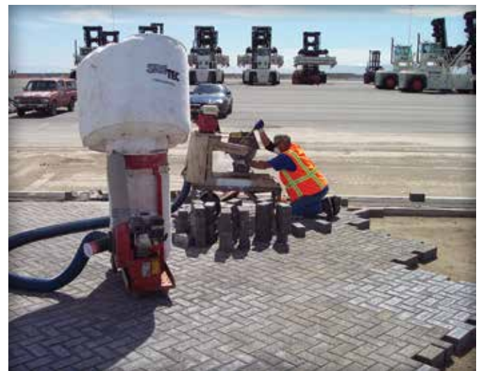
Figure 8. Saw cutting pavers.
