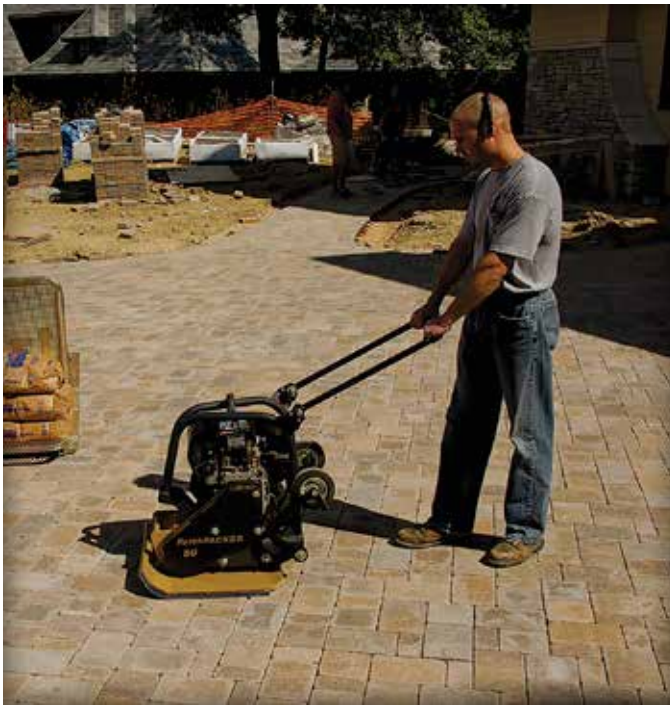
Figure 9. Compacting the pavers and bedding sand.
