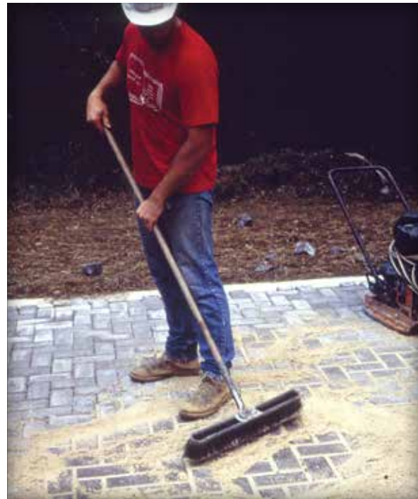
Figure 10. Spreading and sweeping joint sand.
