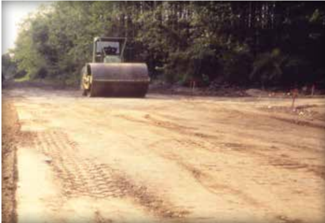
Figure 2. Compacting the soil subgrade.
