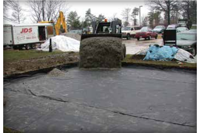
Figure 3. Application of the geotextile under aggregate base.
