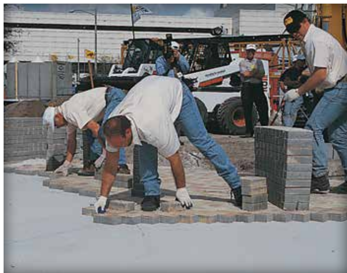
Figure 7. Placing the concrete pavers.
