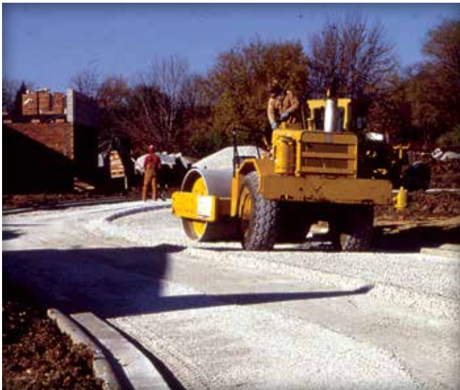
Figure 4. Base compaction with a vibratory roller.
